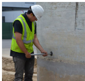
Step 2: Anchor Pin & Mount Guide Post
