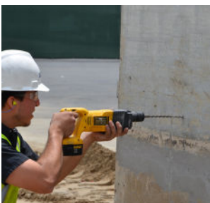
Step 1: Mark Center of Core & Drill Anchor Hole
