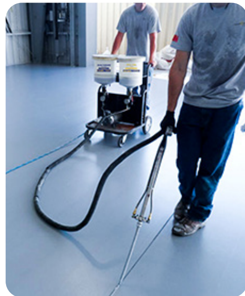
Re-buildable Dispensing Manifold
