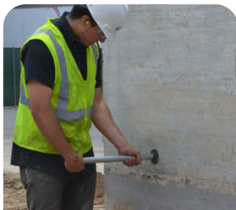
STEP 2: Anchor Pin & Mount Guide Post
