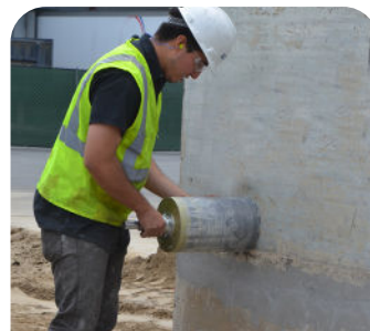
STEP 3: Mount Core Bit Assembly
