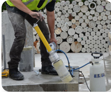
VERTICAL & ANGLED DRILLING
