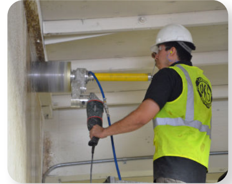
CONFINED SPACE DRILLING
