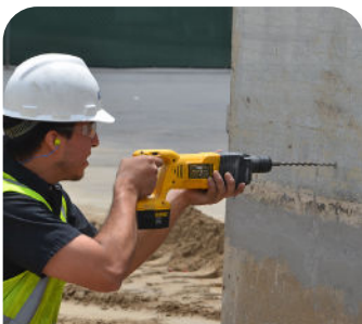
STEP 1: Mark Center of Core & Drill Anchor Hole
