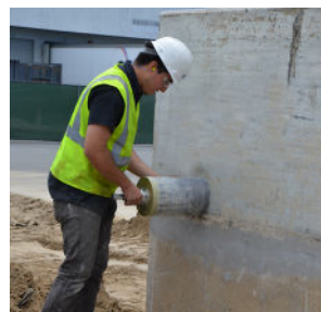
Step 3: Mount Core Bit Assembly
