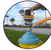
Hydrant Key Available
